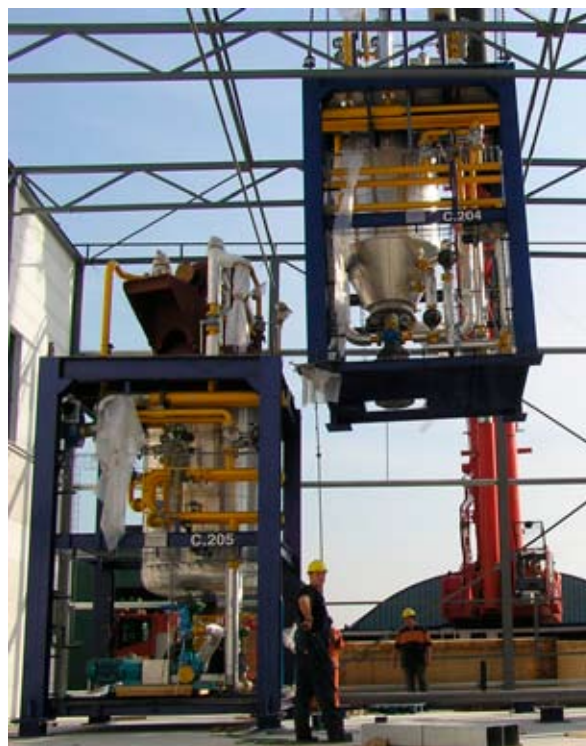
NEW MODULAR GREASE PLANT UNDER CONSTRUCTION AT AXEL'S DUTCH FACILITY
