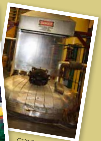
CONTACTOR IN ROSEDALE MISSISSIPPI (USA)
