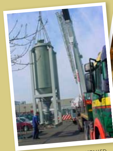
CONTACTOR BEING INSTALLED IN HEIJNINGEN (NL)
